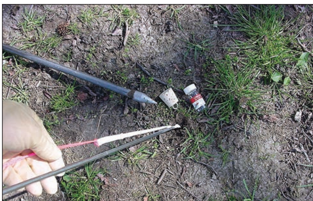
Installation of module in soil.
