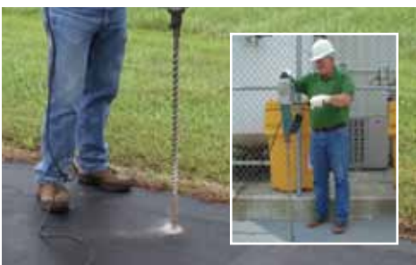
To make hole through slab, use a rotary hammer drill.
