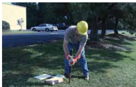
Make a 0.5 –1.0 inch (1 cm) hole 36 in (1 m) deep.
