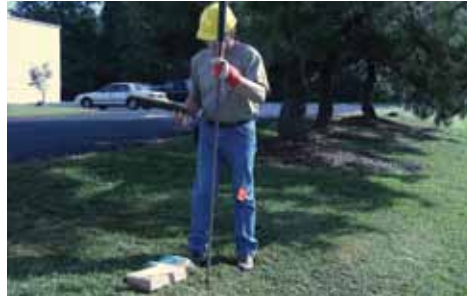
Locate and mark buried utilities and other obstacles.
